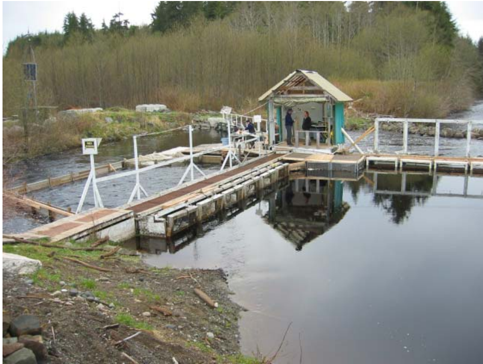
Figure 1. The Keogh River fish fence showing smolt and adult salmon and steelhead trapping facilities, 2002.
